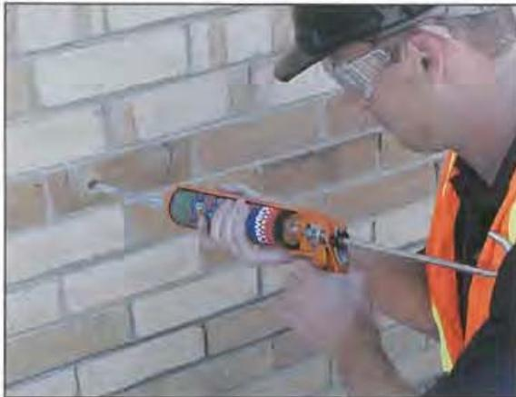
The AC100e (300ml) cartridge system is a versatile, two component, mix in the nozzle, polyester resin system for structural applications. The resin is styrene free and has low odour. The unique 300ml co-axial cartridge system can be used in a standard mastic or professional gun. The operating principle of the tube involves the peeling of the inner tube allowing mixing of the resin and hardener using a static mixing nozzle.
