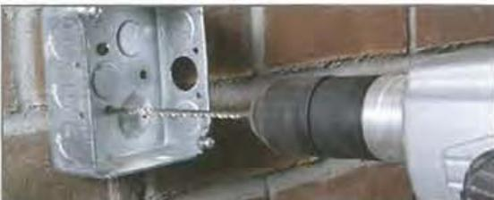
For fixing in concrete, stone or brick pre-drill with a 5mm drill bit.
